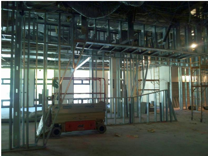
Construction in Progress Sept. 4, 2013
